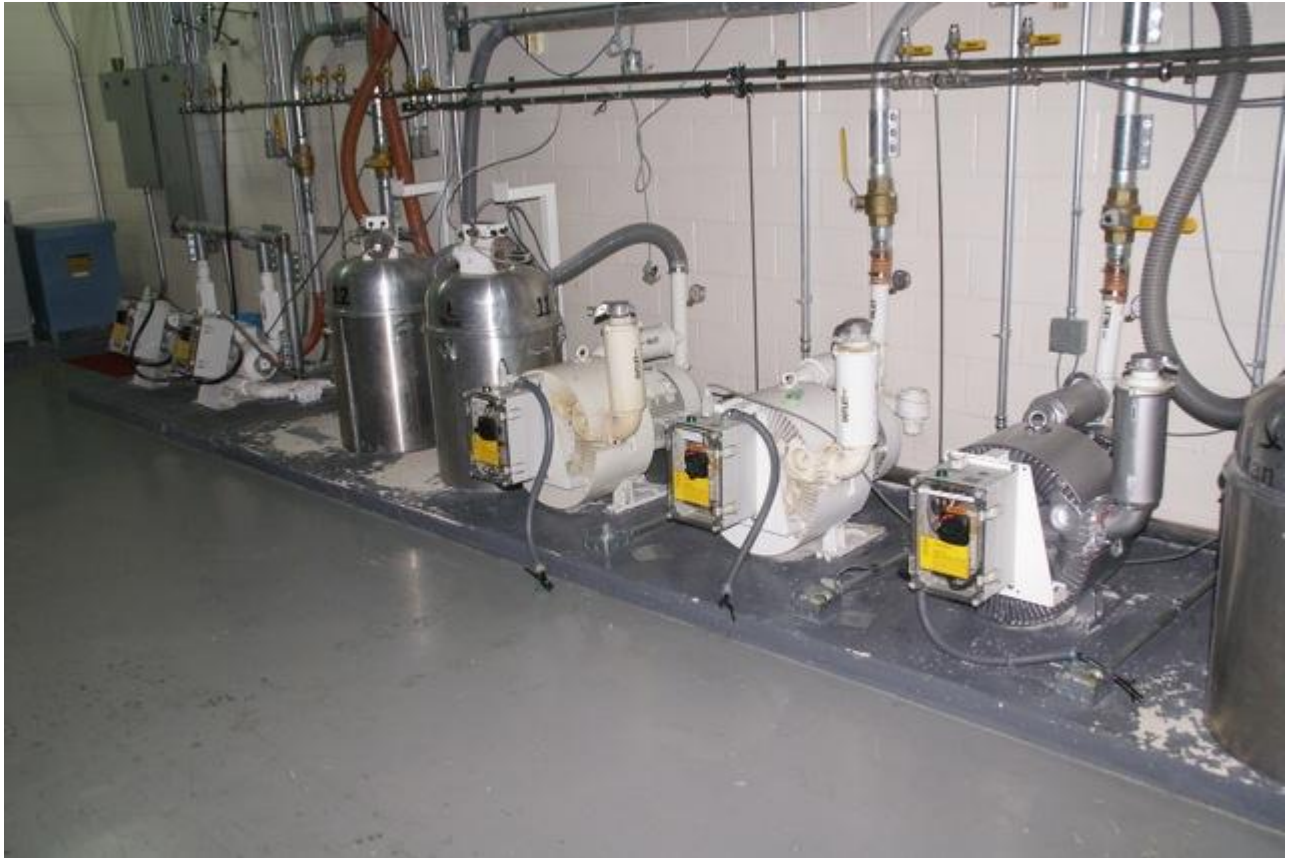
Three (3) 17 hp vacuum blowers, two (2) 6.2 hp vacuum blowers and three (3) pulse filter fines collectors
