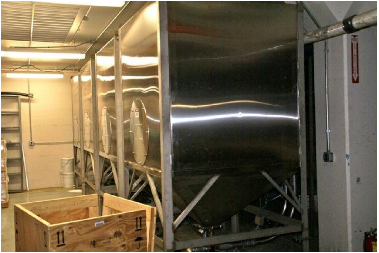
Four (4) storage distribution bins approximately 4,000 il.
