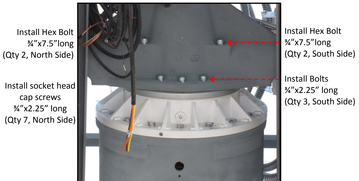
Figure 7 – Install Yoke Hardware (South View)
