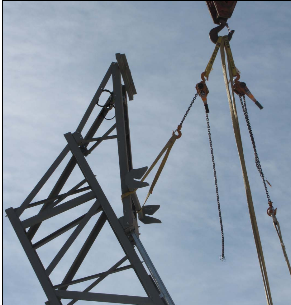
Figure 3 – Install PCU Outer Boom Cross-Bar Tie-Out
