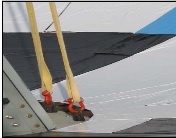
Figure 1 – Install Hub Stabilizer Tie-Out
