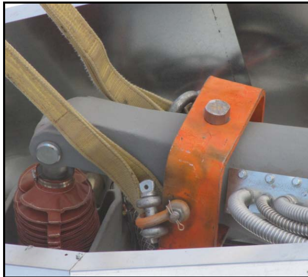
Figure 2 –Yoke Lifting Bracket
