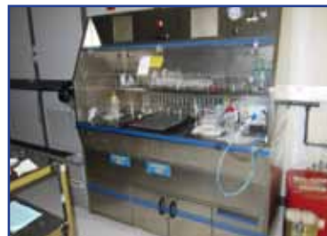
ACID NEUTRALIZATION SYSTEM WITH (2) NEPTUNE MODEL JG 2.10 MIXERS
