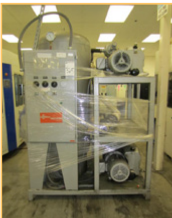
BUSCH VACUUM SYSTEM, WITH RECEIVER TANK
