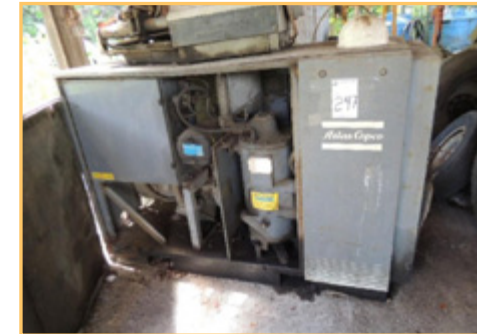
ATLAS COPCO GA-37 AIR COMPRESSOR
