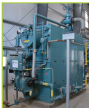
CLEAVE-BROOKS FLX700-800-150ST WATER TUBE BOILER
