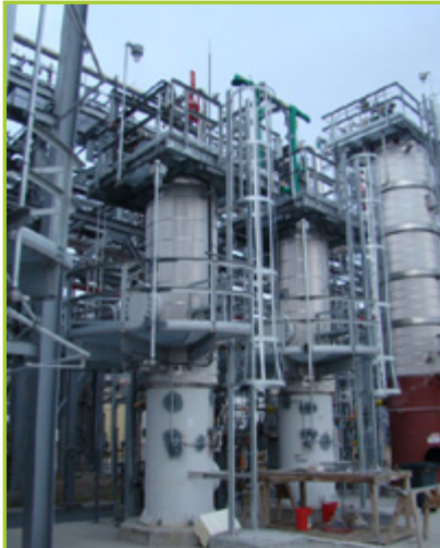
INDUSTRIAL PIPING NB349 STORAGE TANK, 4' X 18'
