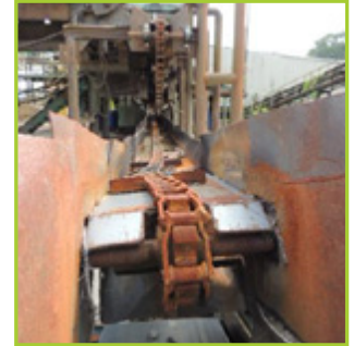
110' STEEL BOX WASTE CONVEYOR
