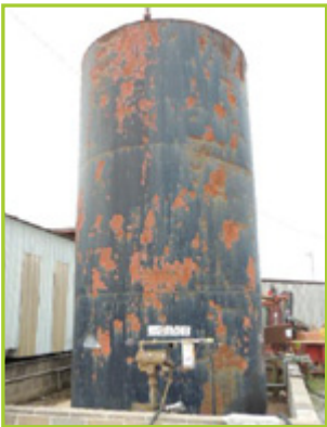
10,000 GAL DIESEL STORAGE TANK
