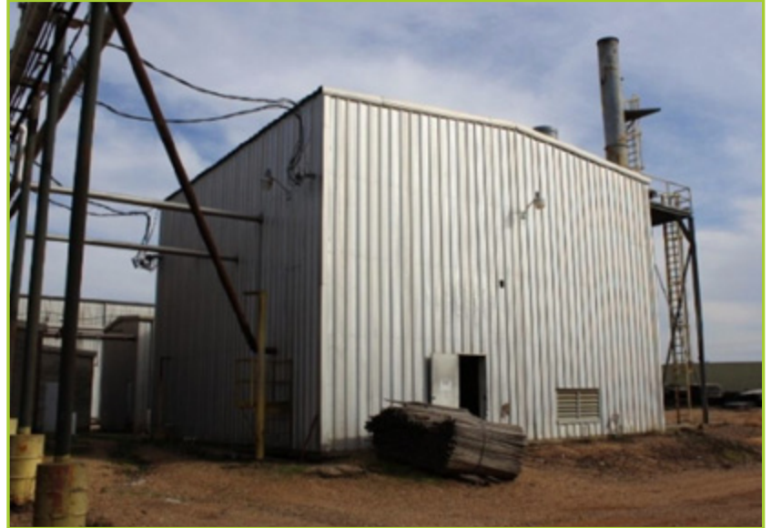
ABCO, WESTINGHOUSE 3076 BOILER BUILDING AND CONTENTS
