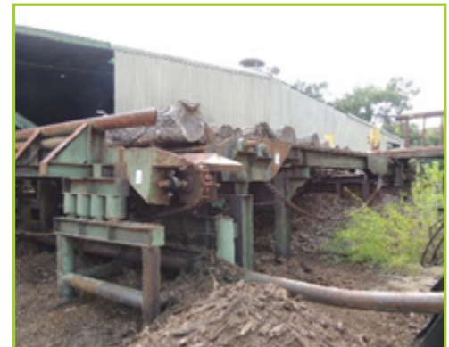
4 STRAND LOG ACCUMULATION DECK
