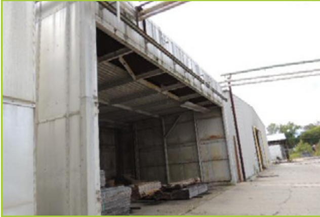
DRY KILN D- AMERICAN WOOD DRYER PACKAGE KILN S, 41 X 34', 75,000 BF CAP
