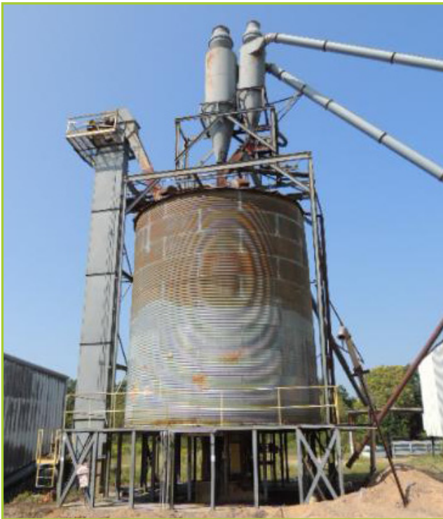
SAWDUST COLLECTION BIN AND 2 CYCLONE BINS
