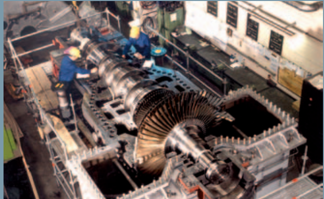
SST-400, Haldia, India; 35 MW. Manufacturing of the condensing turbine at the workshop.
