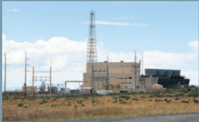
The Blundell Geothermal Plant in Milford, Utah (USA), uses a 26 MW TurboCare condensing turbine with SST-400 GEO steam path.
