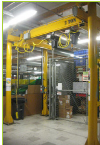
KENDAL OVER HEAD CRANE & KONERANES
