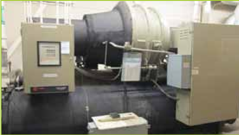
TRANE CVHE450 CENTRAVAC WATER CHILLER
