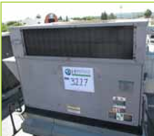
CARRIER 48GSN024040301 3 PHASE PACKAGED GAS HEATING/ ELECTRIC COOLING UNIT
