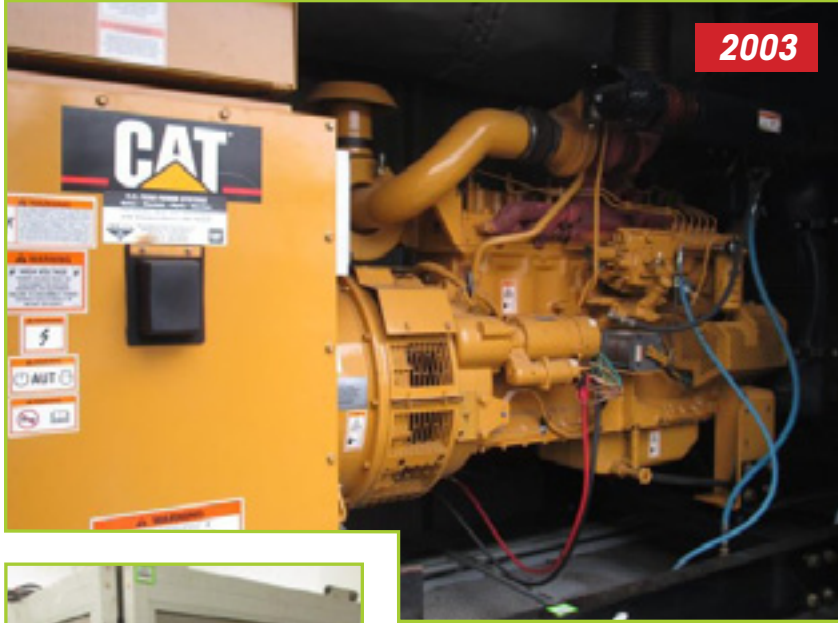
CAT DIESEL GENERATOR, 250 KW, 313KVA, NEW IN 2003, 2 PH, MDL 3306, DIESEL TANK, OUTDOOR ENCLOSURE
