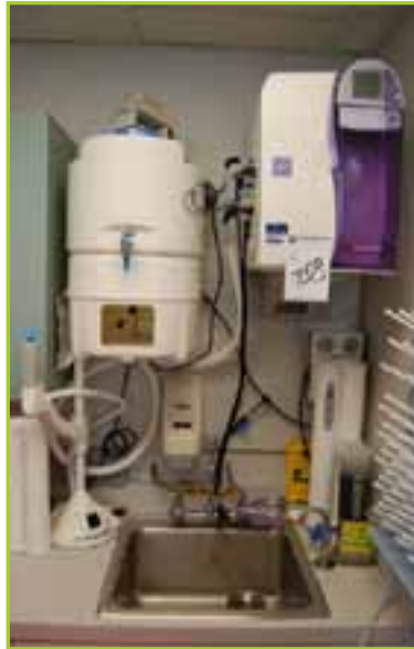
MILLIPORE INTEGRAL WATER SOFTENING SYSTEM
