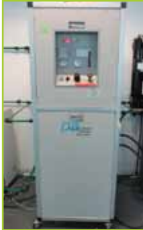
PARKER AGS400NA DUAL BED SERIES NITROGEN GENERATOR
