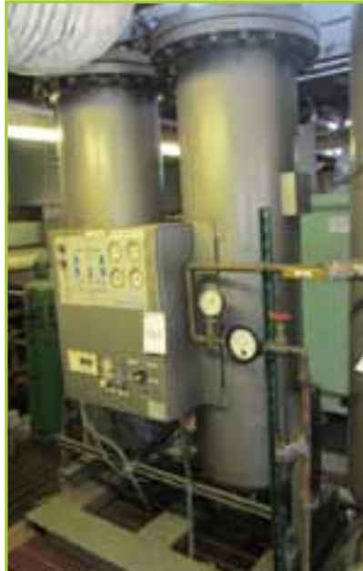
PNEUMATIC 80 NITROGEN GENERATOR
