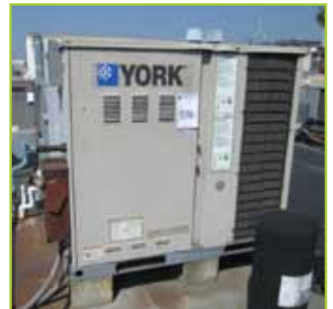
YORK D2NA060N06546D AIR CONDITIONING UNIT
