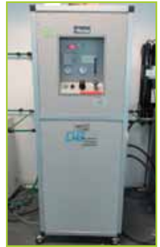
PARKER AGS400NA DUAL BED SERIES NITROGEN GENERATOR
