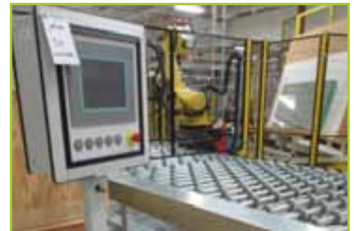
PLC SAFETY SWITCH CONTROLLER CABINET (CABINET FOOTPRINT 7'LX7'HX2'DEEP). INCLUDES: ALLEN BRADLEY LOGIX5563S/LOGIX55SLP PLC SYSTEM ; AB KINETIX-6500/6000 ETHERNET/IP-ENABLED SERVO DRIVER SYSTEM ; AB STRATIX8000 ETHERNET MANAGED SWITCH SYSTEM; ASSORTED AB RELAYS; QTY-1 AB PANELVIEWPLUS-1500 TOUCHSCREEN TERMINAL STATIONS
