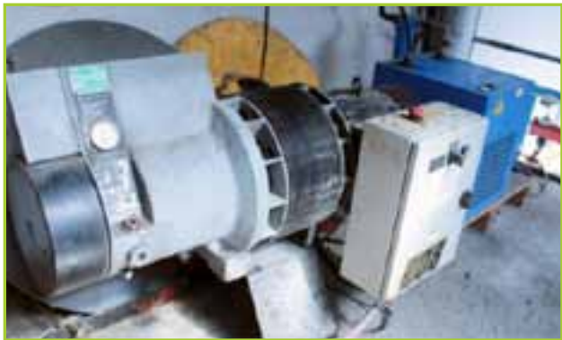
COMPAIR HYDROVANE 43 POWER: 7,5 KW. TOTAL HOURS: 41,680 HR. WITH MTA E800 DRYER AND AIR RECEIVER
