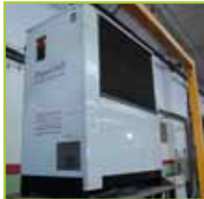
HIROSS HYPERCHILL ICE 010 400/3/50 DHH SINGLE-TOP FAN PACKAGED CHILLER UNIT
