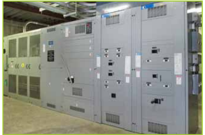
SUBSTATION TO INCLUDE FEDERAL PACIFIC 3 PH, 60 HZ, 500 KVA DRY TYPE TRANSFORMER CLASS AA S/N 11148-001, DISTRIBUTION PANEL WITH (8) SWITCHES, 1,000 AMPS, 3 PH DISCONNECT SWITCH TYPE LCB 15000 VOLTS. (ID# A1 SUBSTATION). LOCATED: GROUND LEVEL, STADIUM INTERIOR. NEAR MEDIA WILL CALL GATE/BY BUS DROP OFF AREA.
