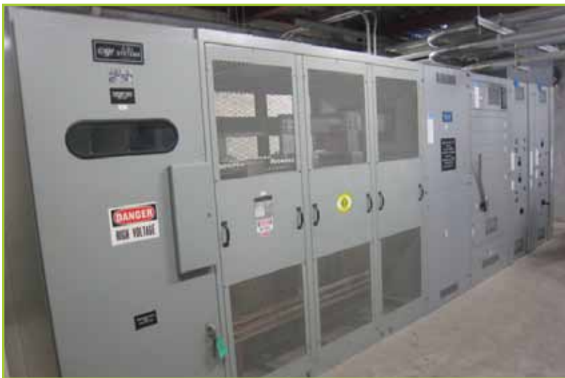
SUBSTATION TO INCLUDE FEDERAL PACIFIC DRY TYPE CLASS AA TRANSFORMER, 3 PH, 300 KVA, S/N 11147-001, GENERAL ELECTRIC 3200 AMPS DISTRIBUTION STATION WITH (7) SWITCHES, HAMMOND POWER 3 PH DRY TYPE TRANSFORMER 208V, 112.5 KVA, P/N NNM112BK
