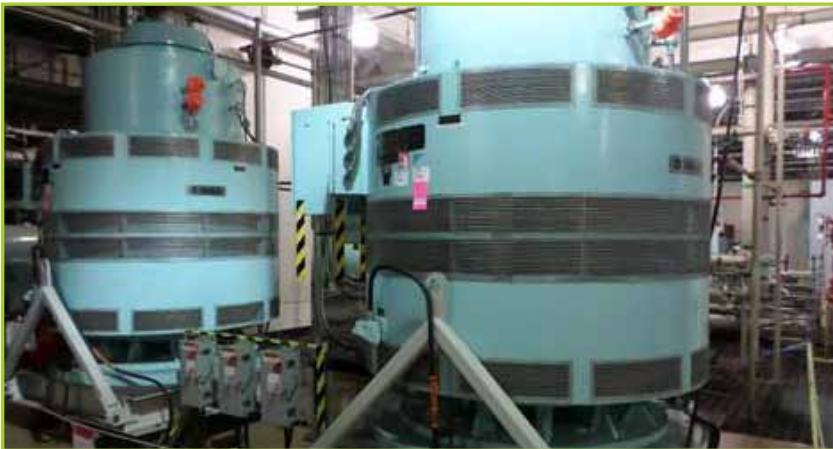
INDUCTION MOTORS GENERAL ELECTRIC 5KV85573446501 LOT TO INCLUDE (2) 2500 HP VERTICAL INDUCTION MOTORS TO INCLUDE MOBILE STANDS
