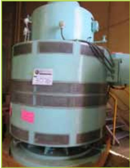
INDUCTION MOTOR GENERAL ELECTRIC 5KV85573446501 INDUCTION MOTOR, PUMP, 2500 HP, 3 PH, 4000V, 60 HZ, 1186 RPM, 8557P70 FRAME, WPII ENCLOSURE, CLASS F INSULATION, 1.15 SF, 315A, NEMA CODE F
