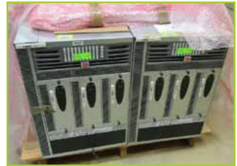
BROCADE 80020207610 SILKWORM 48000 FIBRE CHANNEL (2) SAN SWITCHES
