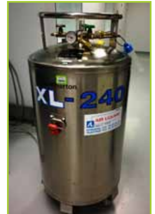
TAYLOR WHARTON LIQUID NITROGEN STORAGE TANK, 250L
