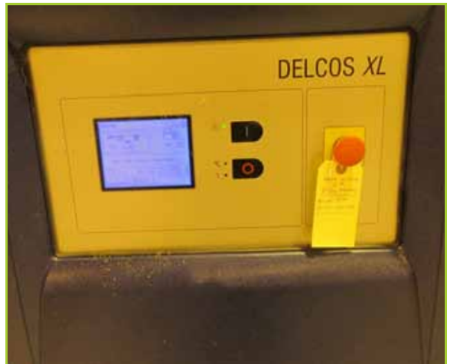
COMPAIR L37RS-13A SCREW TYPE AIR COMPRESSOR , 37 KW MOTOR, 460V, 3 PHASE, 60HZ, DELCOS XL CONTROLS. SN# CD10005426001. YEAR: 2011
