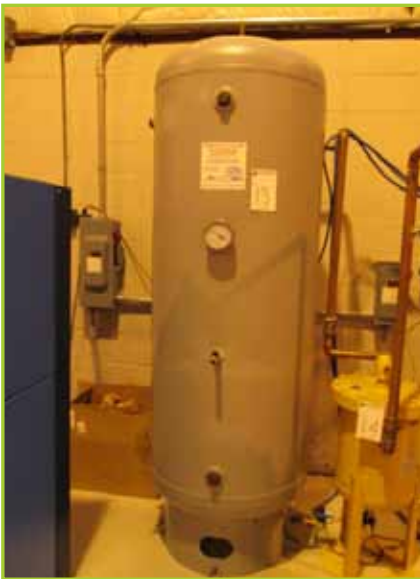
STEEL FAB AIR RECEIVING TANK , MAWP 200 PSI AT 400 DEGREE F, MDMT -20 DEGREE F AT 200 PSI, YEAR: 2011
