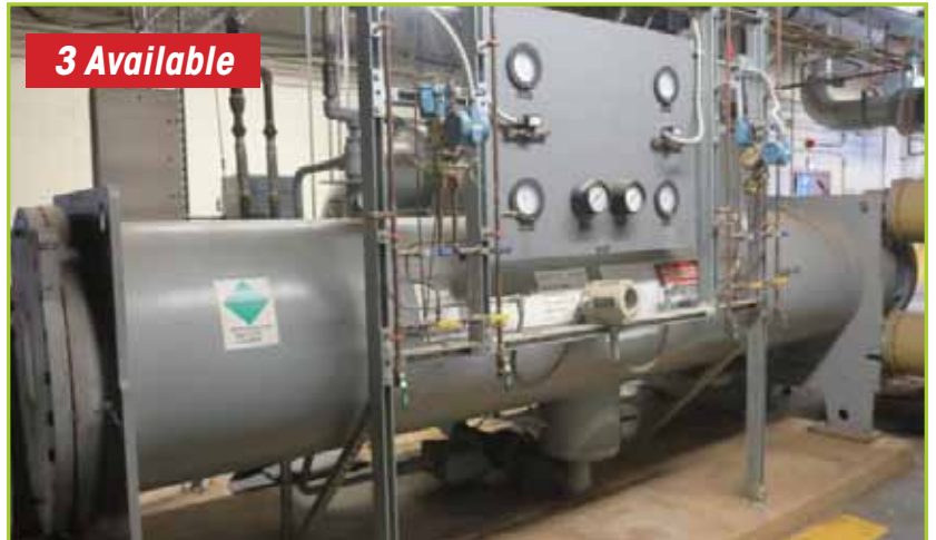
CARRIER / EVERGREEN 19XR INDUSTRIAL CENTRIFUGAL CHILLER
