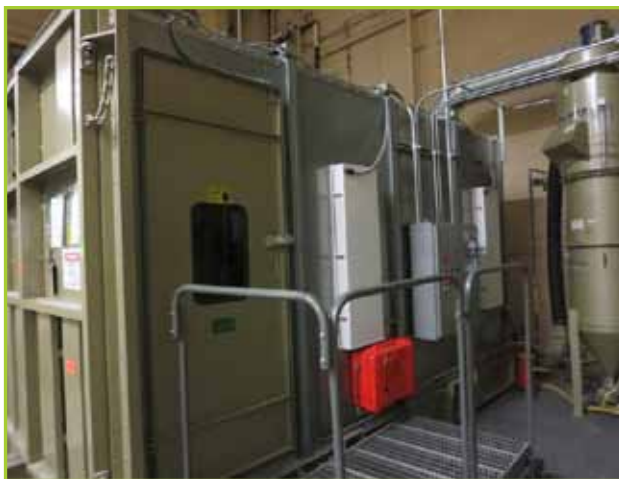
CLEMCO INC., CORP. 7X14X8BLASTROOM ABRASIVE BLAST ROOM
