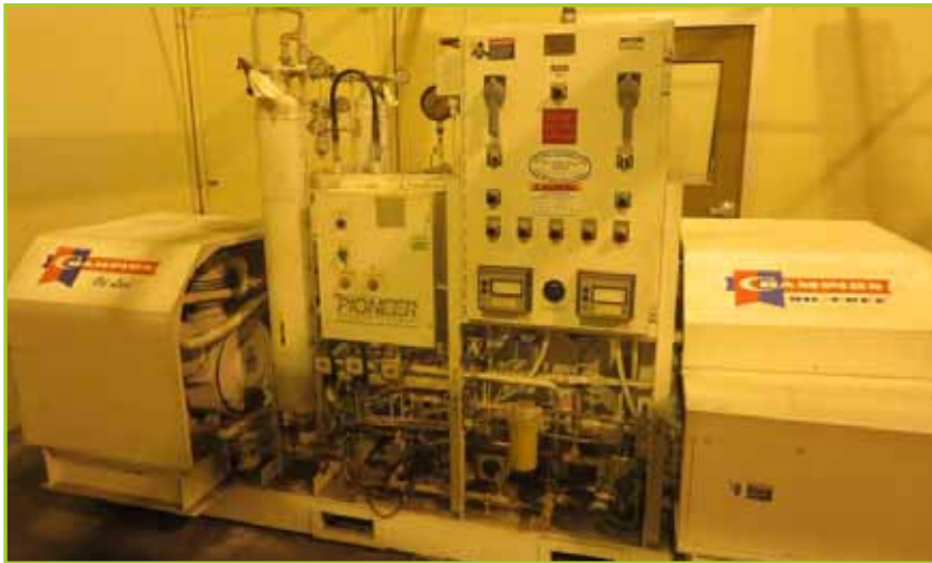
PIONEER PNL 50 COMPRESSOR. 175 PSI WORKING PRESSURE, 200 PSI MAX
