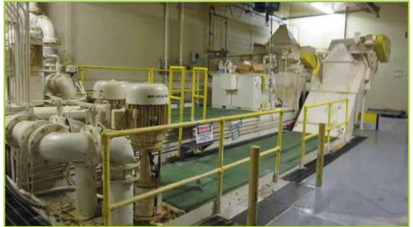
HENRY FILTERS INC 1.800 SID 1-2-12 COOLANT FILTRATION SYSTEM. 4 CIRCULATION PUMPS, 2 TANKS, REFRIGERATION SYSTEM, HENRY FILTERS TANK MIX MODEL 11413-DISO
