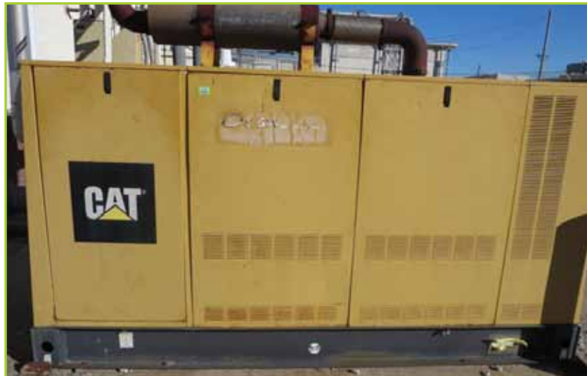
CATERPILLAR 250 KW GENERATOR
