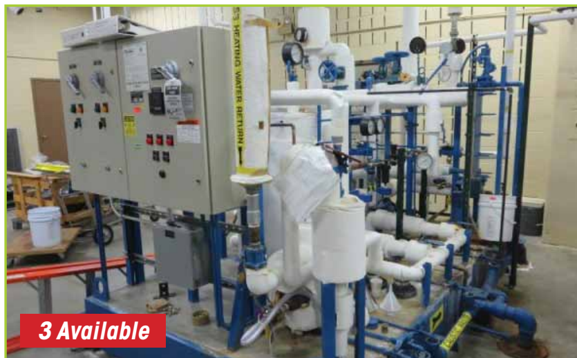
FLO-PAK PCW-101 PROCESSING COOLING WATER SYSTEM. LOT CONTAINS 2 PEERLESS PUMPS 8196 1 1/2 X 8, 71/2 HP 3500RPM STAINLESS STEEL. 20 GPM AT 230'
