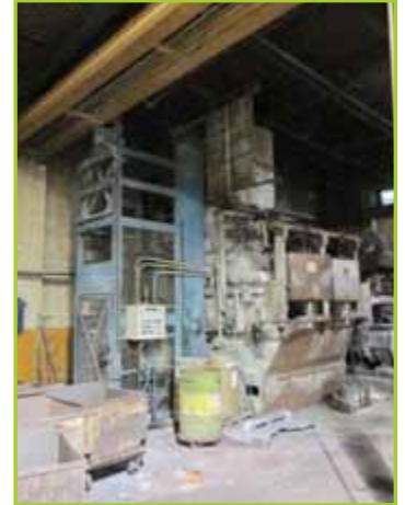
STRIKO PA15480 FURNACE
