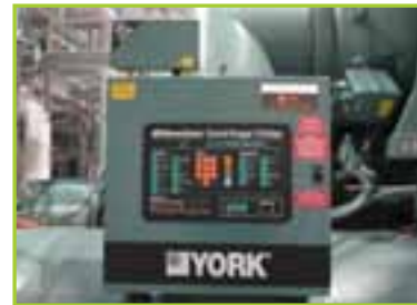
(2) YORK YTL6D8F2-CWH CHILLER SYSTEM, R123, COMPRESSOR MODEL YTDL-144
