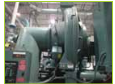
(2) YORK YTL6D8F2-CWH CHILLER SYSTEM, R123, COMPRESSOR MODEL YTDL-144
