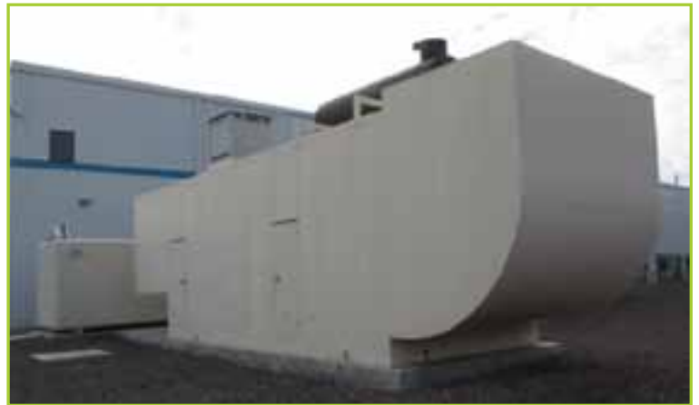
(2) YORK YTL6D8F2-CWH CHILLER SYSTEM, R123, COMPRESSOR MODEL YTDL-144
