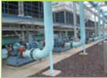
EVAPCO USS 228-0824 QTY (3) 2 TON COOLING TOWERS , 30,000.000 CAPACITY (MBH), 6,000 GPM, AIR FLOW CFM 427,800 PER UNIT, WET BULB (F) 78, (6) VARIOUS ELECTRIC MOTORS, (6) ALLIS-CHALMERS PUMPS 3000 GPM, (2) ABB 550 VFD (4) ABB 500 VFD, STORAGE CABINETS AND SUPPORT EQUIPMENT
