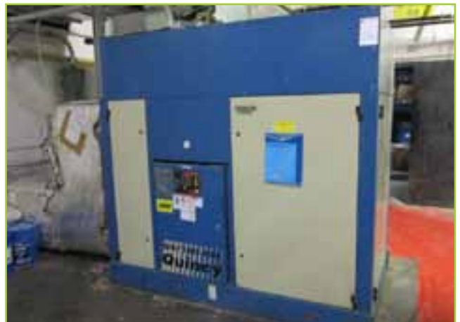
QUINCY ROTARY QSF150-125 SCREW AIR COMPRESSOR
