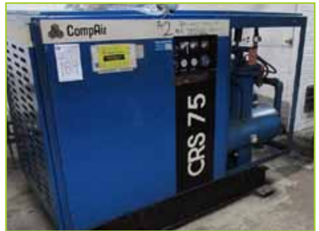
COMP AIR CRS75 COMPAIR ROTARY AIR COMPRESSOR, 75-HP
