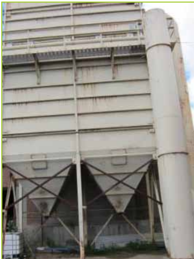
(2) CHUTE SAND SILO WITH STRUCTURE
