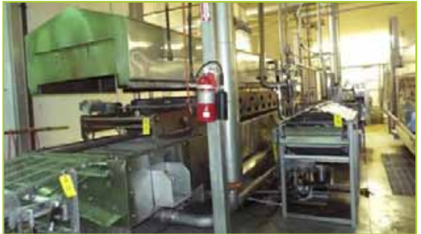
HEAT & CONTROL FRYER, MODEL BPF, PROJECT# 2003004520, 460 VOLTS, 6.6 AMPS, 3 PHASE 60 HZ, WITH CORNELL DUMP, FILTER, HEXCHANGER & HOLD TANK, 37 IN. BELT, 28 FT. LONG
