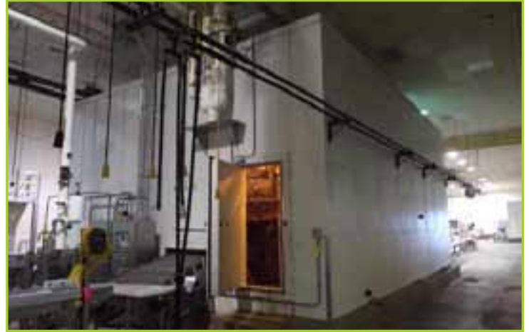
NORTHFIELD DUAL BELT SPIRAL FREEZER 30 IN WIDE BELT, 3 IN. CLEARANCE, 20 LEVELS, 10 PER LINE, BOTTOM INFEED, TOP DISCHARGE, BOLTED DESIGN, ACTIVE BELT LENGTH 1000 FEET
