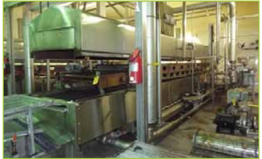
HEAT & CONTROL FRYER, MODEL BPF, PROJECT# 2003004520, 460 VOLTS, 6.6 AMPS, 3 PHASE 60 HZ, WITH CORNELL DUMP, FILTER, HEXCHANGER & HOLD TANK, 37 IN. BELT, 28 FT. LONG
