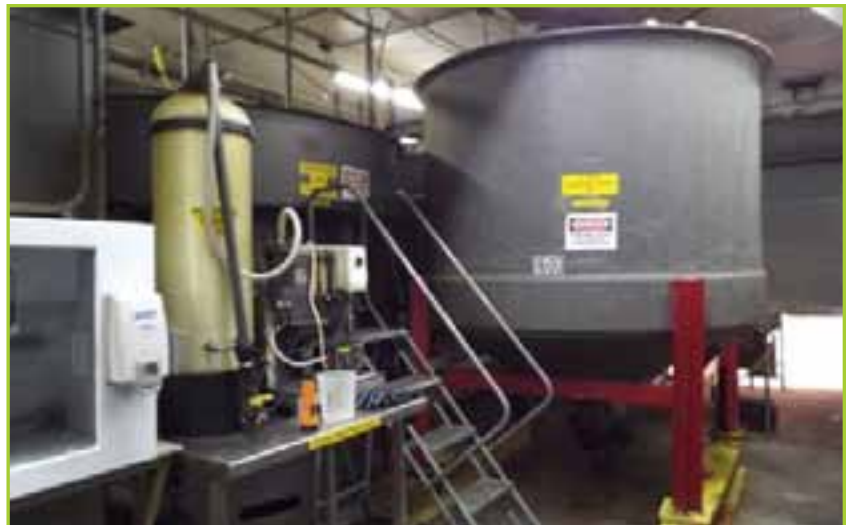
ANDERSON NICKLES DAF WASTE WATER TREATMENT SYSTEM INCLUDES 45,000 GALLON EQUALIZATION TANK, (2) 11,000 BIO TANKS, DAF UNIT, TRANSFER PUMPS, ROTO STRAINER, WASTE SCREW CONVEYOR AND SLUDGE CONTAINER
