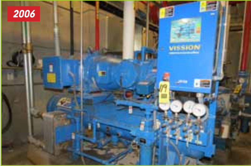
2006 VILTER 125 HP SCREW AMMONIA COMPRESSOR, MODEL: V5M361, S/N: 4145, WITH VISION MICROCONTROLLER AND RAM STARTER
