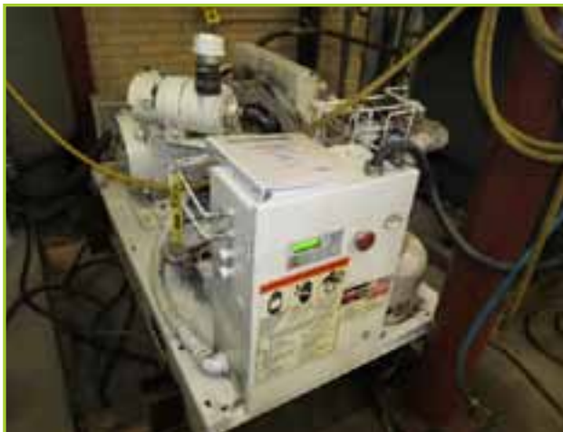
GARDNER DENVER 30 HP SCREW AIR COMPRESSOR
