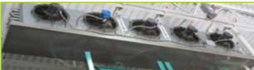
(19) 2006 VILTER AMMONIA BLOWERS
