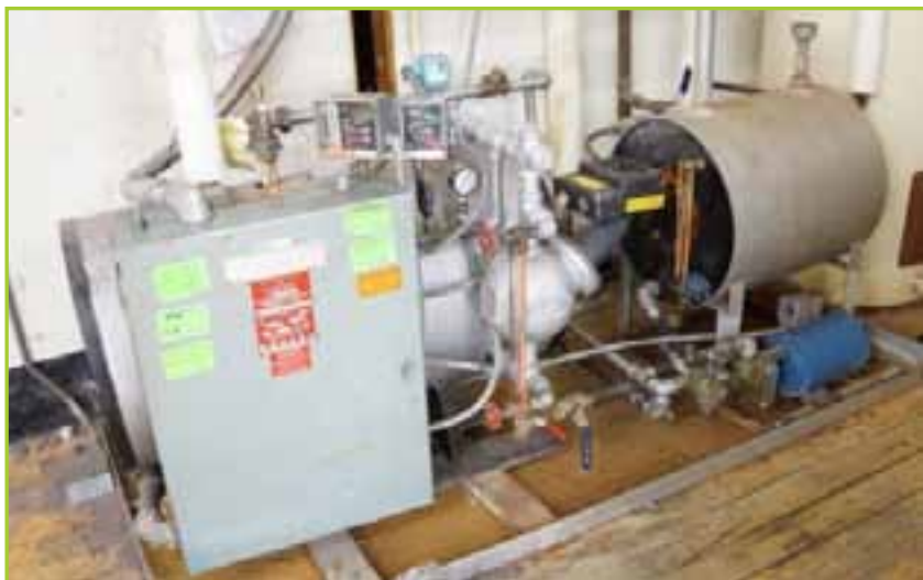
REAMERS ELECTRIC STEAM BOILER RH35 36 KW 220 VOLTS 3 PH 60 CYCLES
