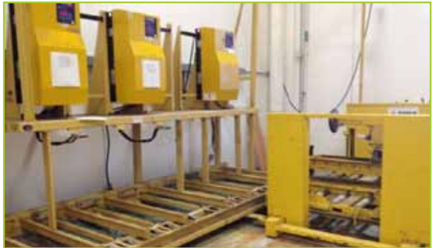
FORKLIFT BATTERY CHARGING STATION WITH LOADER
