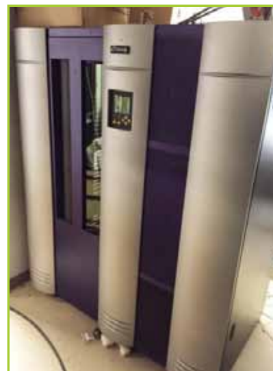
STORAGETEK L700E LTO-3 DIGITAL TAPE LIBRARY WITH 416 SLOT CAPACITY W/(2) TAPE DRIVES
