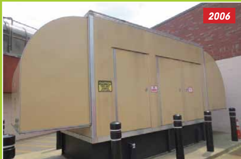
CATERPILLAR A.A. PACKAGED GENERATOR SET. ENGINE C27 S/N DWB00.166/MJE00100, GENERATOR SR4B S/N AFH00594. 700KW. 277/480 V. 2006. 209.5 HOURS. WITH 2 CAT ENTELLI-SWITCH 250 SWITCHES. 2- 300KVA TRANSFORMERS
