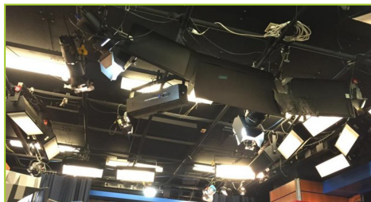
26'X18.5' SET W/LIGHTING GRID, (1) VIDESSENCE P110-255BX, (8) ENTERTAINMENT TECHNOLOGY IPS-DS-1206, (2) ETC DESIRE D40, (2) ETC SOURCE FOUR JR., (1) PEPPER 200, (3) VIDESSENCE 650L FRESNEL, (1) ARRI LED, (1) ARRI 650 PLUS, (1) MOLE RICHARDSON 3131 MOLEQUARTZ. (1) PHILLIPS STRAND 200 PLUS DMX CONTROLLER, (1) AOC E90S MONITOR
