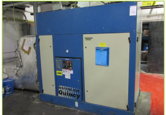
QUINCY ROTARY QSF150-125 SCREW AIR COMPRESSOR
