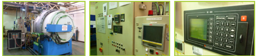
ALD VKA 60/60/90 VACUUM TEMPERING FURNACE RATED TEMP 750DEGC, WORKING CAP 90KW, 440V, 50HZ, 168A, CONTROL CABINETS & PANELS, DIGITAL & ANALOGUE CHART RECORDERS, DIGITAL OVEN CONTROL PANEL, STANGE SE404 DIGITAL MONITORING PANEL - YOM 2000
