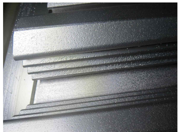
Figure 5. Row 2 Dovetail Pitting
