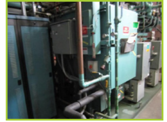
STOKES 264 SQ. FT. FREEZE DRYER. CHAMBER MAWP 18PSI @ 260°F, MDMT -20°F @ 18PSI 2 SKIDS, REBUILT IN 2008, CONDENSER YR 2003 & REFRIGERATION (2) COPELAND 6TM1-2000-TSK-800 COMPRESSORS. UP GRADED CONTROLS WITH OLD CONTROLS FOR BACKUP.
