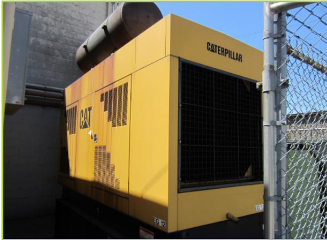
CATERPILLAR 3406 DIESEL 350KW GENERATOR. 893HRS. MFG. YR: 2000
