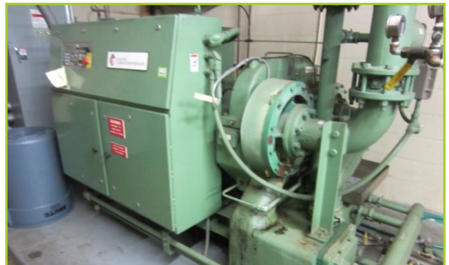
COOPER TURBO COMPRESSOR TURBO AIR 2000 AIR COMPRESSOR. 150HP, 125PSIG
