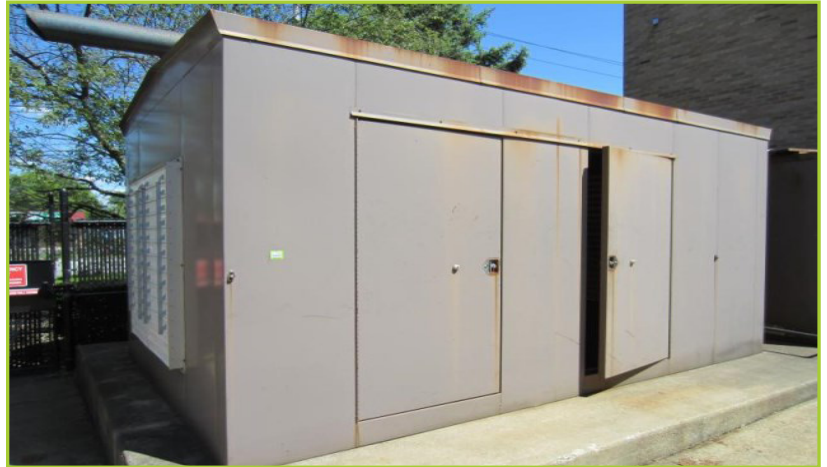
CATERPILLAR G3406 NATURAL GAS 250KW GENERATOR. HRS 810, CATERPILLAR ENGINE MODEL 3406
