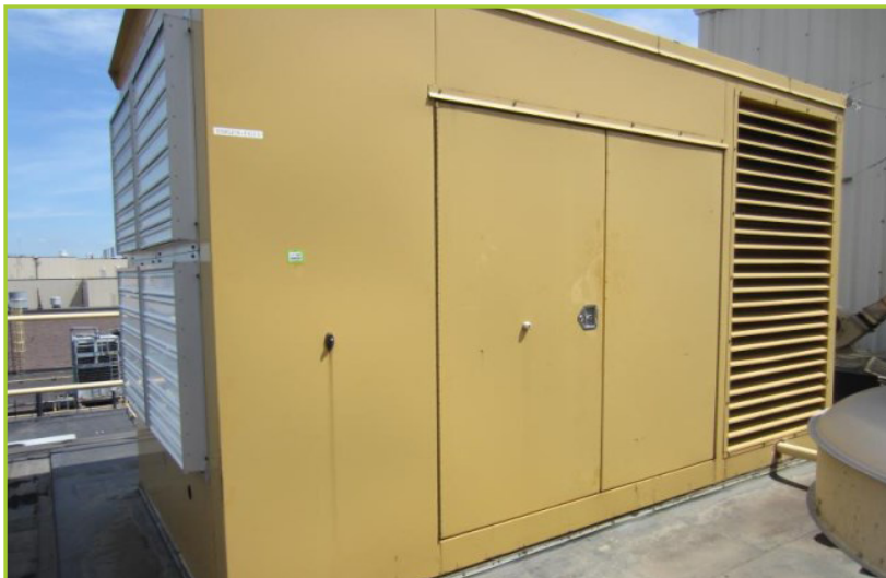
CATERPILLAR G3406 255KW NATURAL GAS GENERATOR. 318KVA. WITH TRANSFER SWITCH, EMERSON ASCO 7000 SERIES POWER TRANSFER SWITCH
