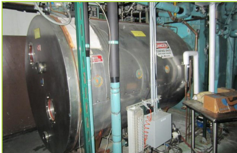
STOKES 360 SQ FT. FREEZE DRYER. REBUILT IN 2008. CHAMBER MAWP 18PSI @ 260°F, MDMT -20°F @ 18PSI, 2 SKIDS, CONDENSER YR 2003 & REFRIGERATION. UP GRADED CONTROLS WITH OLD CONTROLS FOR BACKUP
