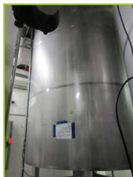
16,500 LITER STAINLESS STEEL TANK. VESSEL VOLUME 5000GAL, VESSEL M.A.W.R.50-15 PSI @350°F, NATIONAL BOARD # 4627. 8'6" DIA X 11' .500THK 316L STEEL YR 2000 NON JACKETED.YEAR: 2000
