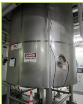
16,500 LITER STAINLESS STEEL TANK. VESSEL VOLUME 5000GAL, VESSEL M.A.W.R.50-15 PSI @350°F, NATIONAL BOARD # 4626. 8'6" DIA X 11' .500THK 316L STEEL YR 2000 NON JACKETED.YEAR: 2000
