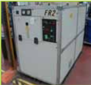
HIROSS HYPERCHILL ICE 010 400/3/50 DHH SINGLE-TOP FAN PACKAGED CHILLER UNIT, YEAR: 2003
