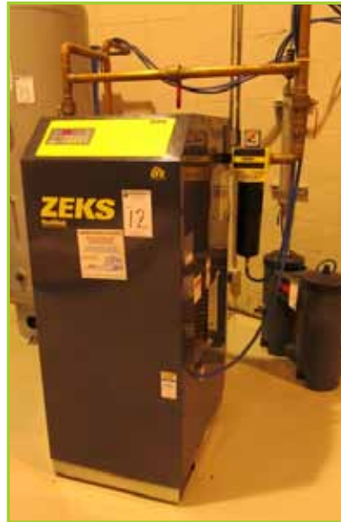
ZEKS HEAT SINK 250HSGA400 TRUE CYCLING AIR DRYER , 300 PSIG, YEAR: 2011
