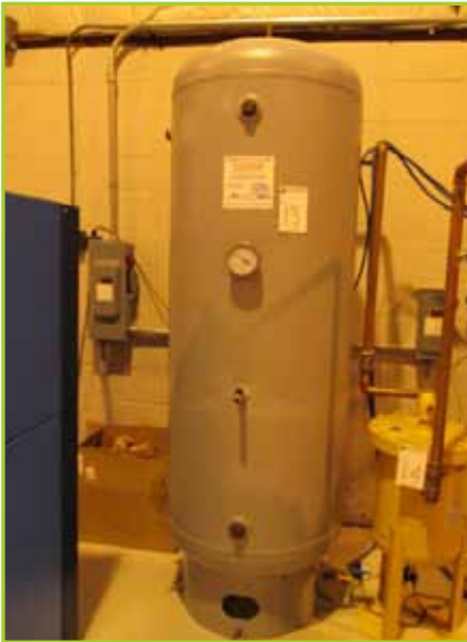
STEEL FAB AIR RECEIVING TANK , MAWP 200 PSI AT 400 DEGREE F, MDMT -20 DEGREE F AT 200 PSI, YEAR: 2011
