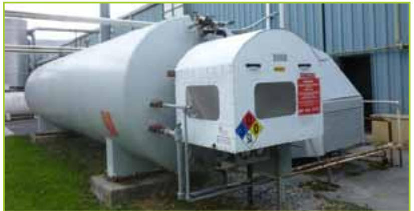
(2) CO2 TANKS, 30 TONS EACH CO2 VAPORIZER, MOUNTED ON WALL 150' CRYOTECH NITROGEN 5/8" PIPING
