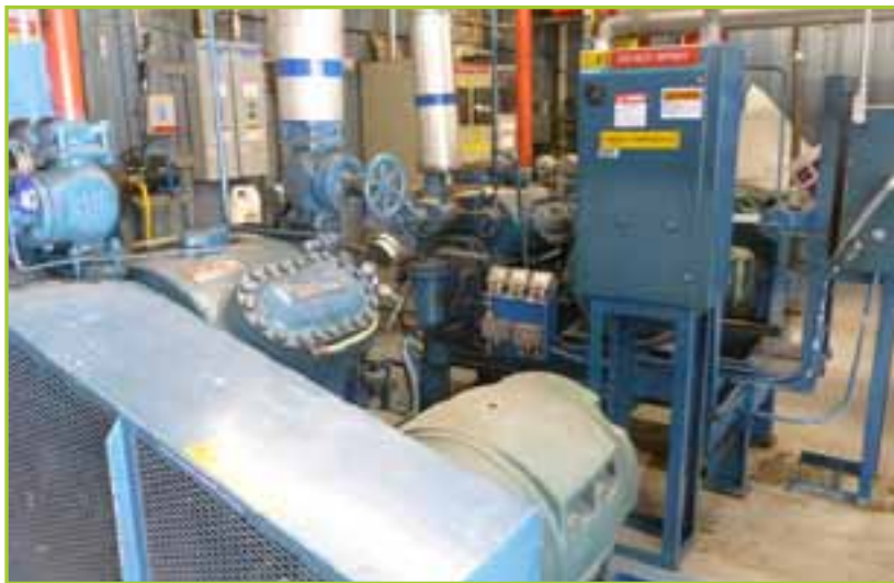
(2) VILTER VMC 450 XL 8-CYLINDER 150HP RECIPROCATING COMPRESSORS
