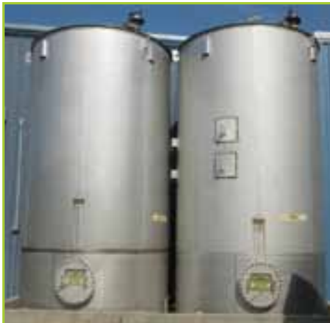
(2) BENDEL 10,000 GALLON SINGLE SHELL 316L S/S SYRUP TANKS
