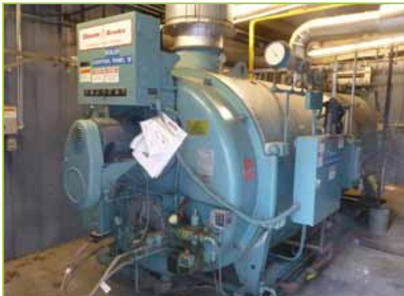
CLEVER BROOKS NATURAL GAS BOILER, MODEL: CB200200015, S/N: 0109973, RETUBED 2008, 200HP, 15 PSI, WITH WATER MAKE UP SYSTEM, WATER SOFTENER, US FILTER, UV LIGHT
