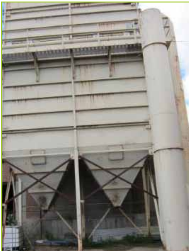
(2) CHUTE SAND SILO WITH STRUCTURE
