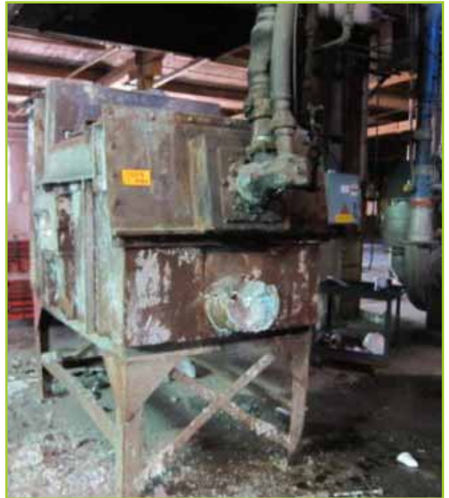
LIQUID NITROGEN TANK, 10626
