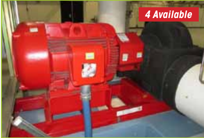
BELL AND GOSSETT 2100 10X12X12M SERIES CENTRIFUGAL PUMP HSC3 WITH 150 HP BALDOR MOTOR, ABB 550 VFD AND GE SAFETY SWITCH
