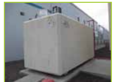
CATERPILLAR 3516 2000KW DIESEL GENERATOR , ENGINE HOURS 22, S/N GZS00628, GENSET MODEL SR4B S/N 8NN01288 YR 2006, 5000 GAL TANK WITH OLDCASTLE CONVAULT MODEL RN 5000 3S TANK ENCLOSURE
