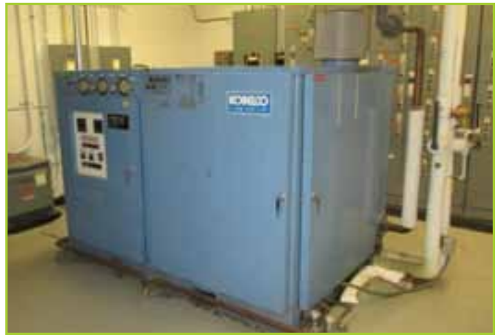
KOBELCO KNW1-A 100 HP ROTARY SCREW AIR COMPRESSOR
