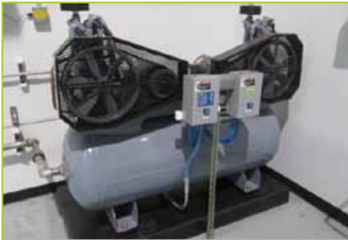
GARDNER DENVER R-SERIES COMPRESSOR , CADRSA, R SERIES 1.5-30 HP, S/N DM015286
