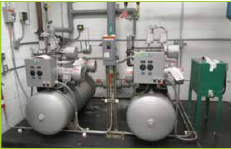
BUSCH RC0100E.506.1003 VACUUM SYSTEM, (2) TYPE R5, ROTARY VANE PUMPS, 63 CFM @ 15 TORR, (2) 5 HP TOSHIBA PUMPS PER TANK, S/N 105373, WITH MOTIVAIR .AC0100 AIR CHILL UNIT
