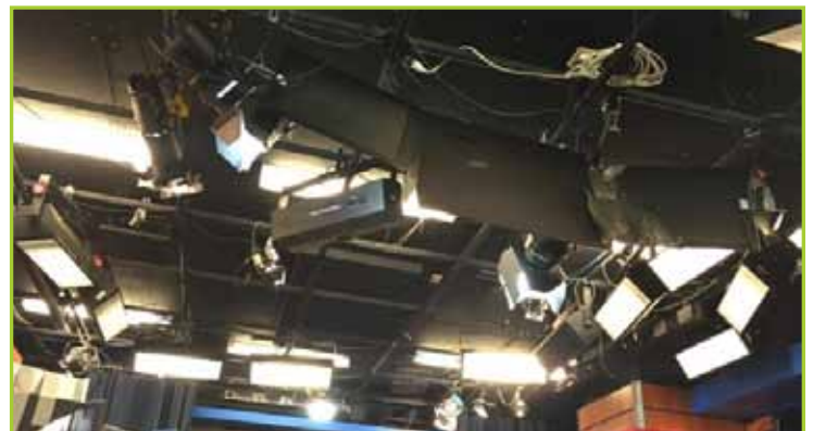
26'X18.5' SET W/LIGHTING GRID, (1) VIDESSENCE P110-255BX, (8) ENTERTAINMENT TECHNOLOGY IPS-DS-1206, (2) ETC DESIRE D40, (2) ETC SOURCE FOUR JR., (1) PEPPER 200, (3) VIDESSENCE 650L FRESNEL, (1) ARRI LED, (1) ARRI 650 PLUS, (1) MOLE RICHARDSON 3131 MOLEQUARTZ. (1) PHILLIPS STRAND 200 PLUS DMX CONTROLLER, (1) AOC E90S MONITOR
