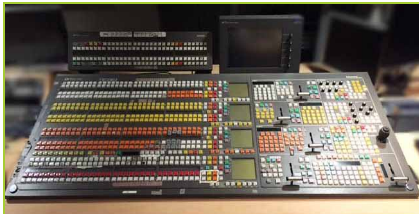
GRASS VALLEY KALYPSO 4 M/E PRODUCTION SWITCHER (M/E 1 HAS FAULTY CARD)
